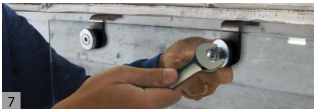
7 Holding the glass panel in place, assemble the outer Chloroprene washers and steel rings, then tighten securely.
