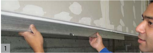
1 Verify that the supporting construction is level.
