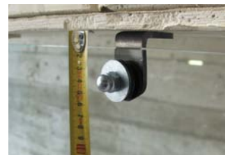
8 Verify perimeter gaps (a to f) and alignment of the glass panels, adjust as necessary.
