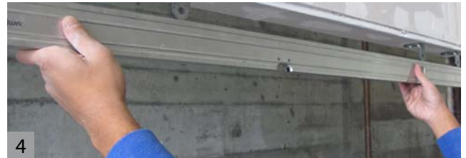
4 Verify that the brackets are level, shim as required.
