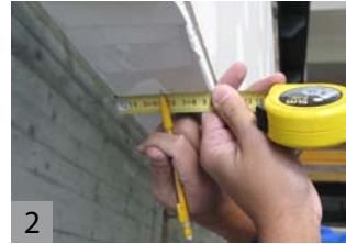
2 Locate the fixing points of the brackets on the supporting construction (concrete or lightweight partition).
