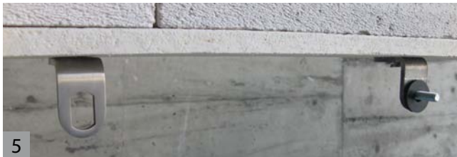
5 Prepare the brackets placing the Chloroprene washers onto the bolts, (fasteners and washers are supplied with the kit).
