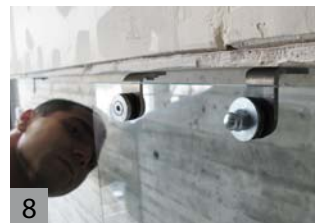
8 Verify perimeter gaps (a to f) and alignment of the glass panels, adjust as necessary.
