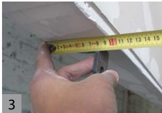
3 Check the alignment of the brackets.
