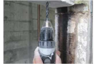
2 Locate the fixing points of the brackets on the supporting construction (concrete or lightweight partition).
